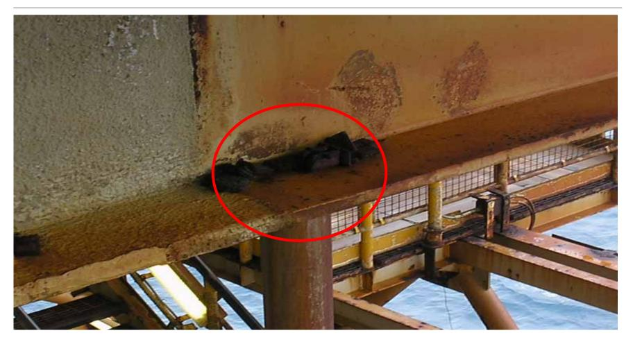
Redundant clamps left on beam – Unsecured Drops Hazard (Clamps were removed from beam after photo was taken)
