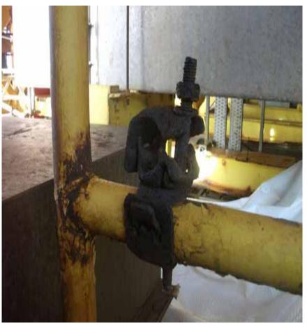
A redundant handrail and scaffolding clamp left in place for some time.
